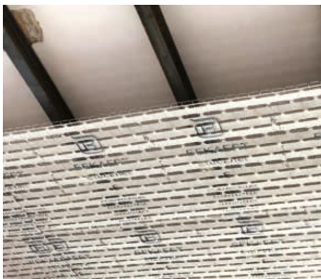
SISTEMA X PLASTER: FORMAZIONE SECONDO STRATO INTONACO PLASTERWALL.
